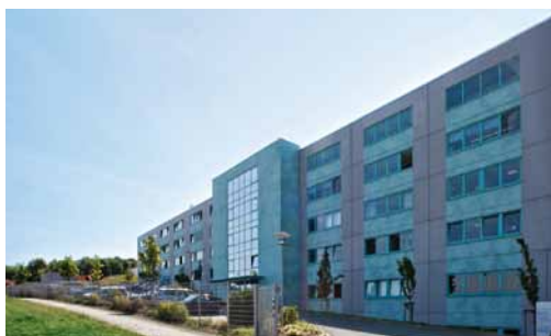
New state-of-the-art production site in Schalksmühle, Germany
